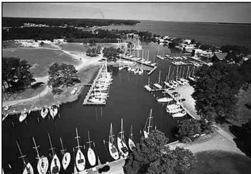
Figure 3. Aerial photograph of Stingray Harbor Marina.
